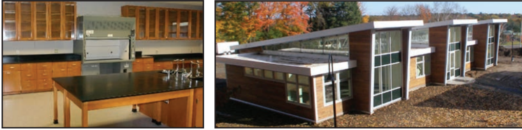
Figure C.3 Examples of Prefabricated Science Classrooms
